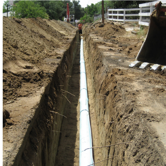
Environmental Infrastructure Loans
